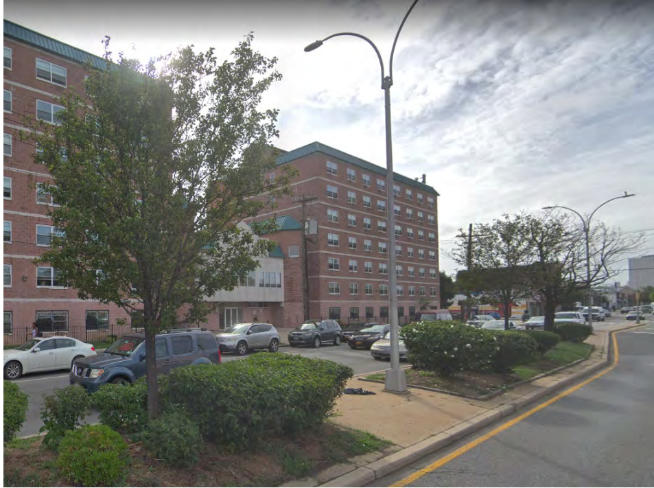
Photo 9-11: View of NYC Greenstreets property median looking northwest from Merrick Boulevard. Allen Cathedral Senior Residences are visible in the background.
