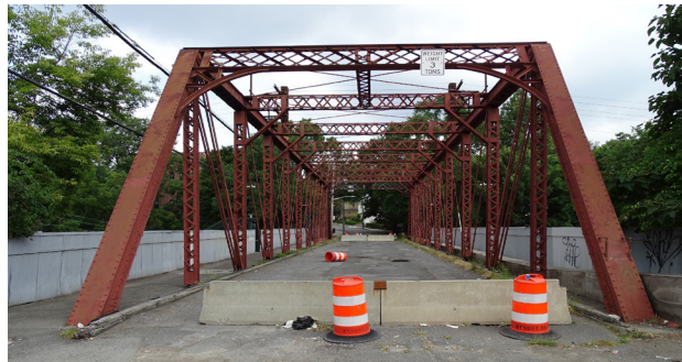
Fulton Avenue Bridge in Mt. Vernon
