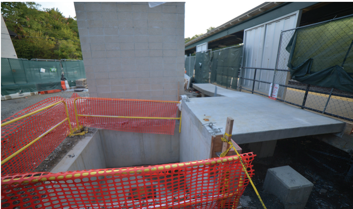
Crews prepare Hartsdale Station for a new elevator and accessibility improvements
